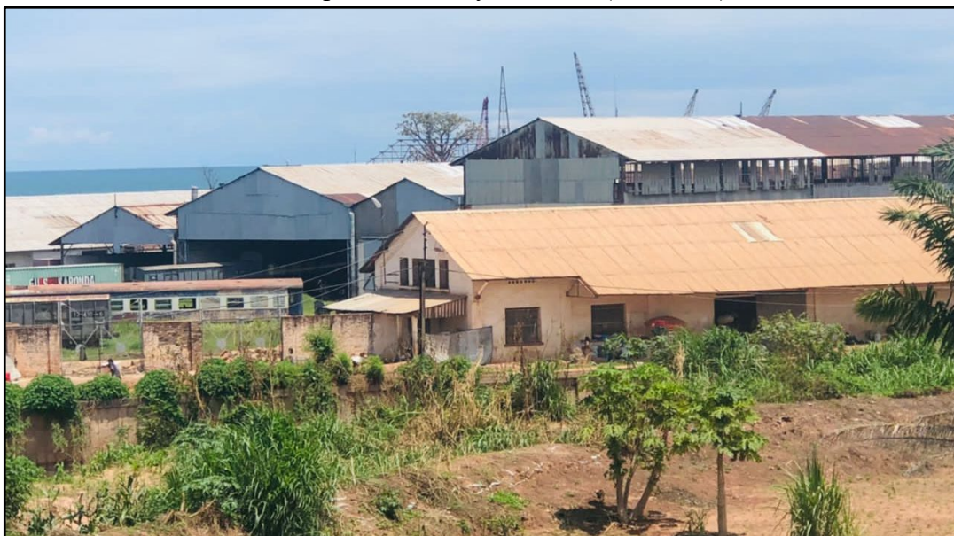
Figure 3: Warehouse at Kalemie Port © Octopus Consulting & Insight
