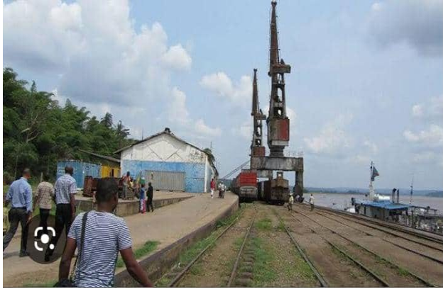
Figure 6: Train Station in Ilebo (Kasai)
